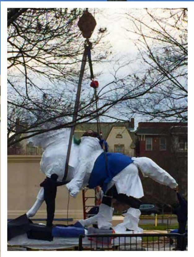
Installation of the horse and rider took place on December 6, 2019
